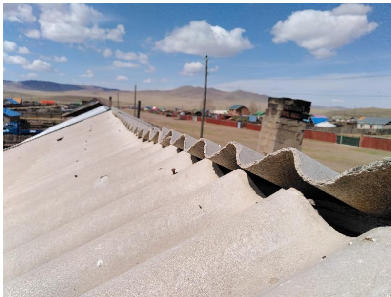
Example of a roof with asbestos
