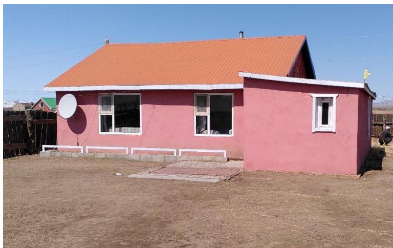
Example of a house made by hollow concrete blocks
